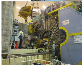
ARICH+FWD ECL installation
