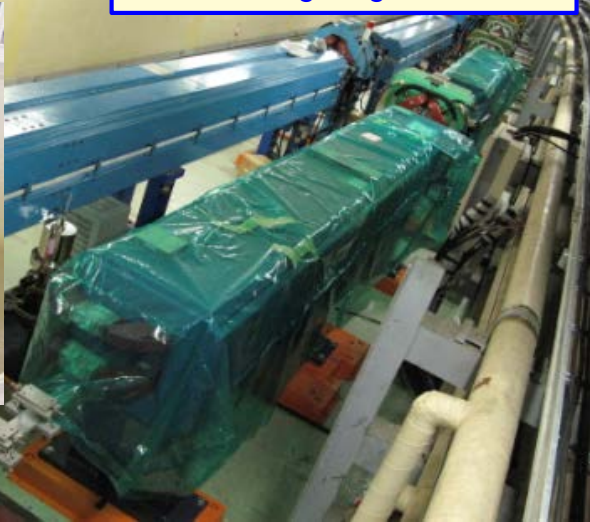
Installation of 100 new long LER bending magnets
